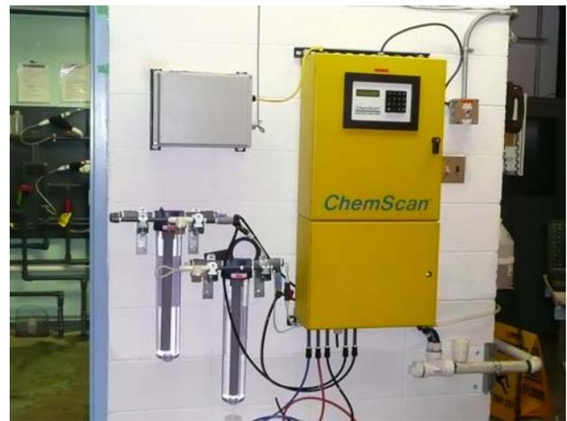
*The ChemScan UV-2150/S Chloramination Analyzer is the only Analyzer capable of monitoring all four key parameters, Monochloramine, Free Ammonia, Total Ammonia and Total Chlorine from two sample points.*
